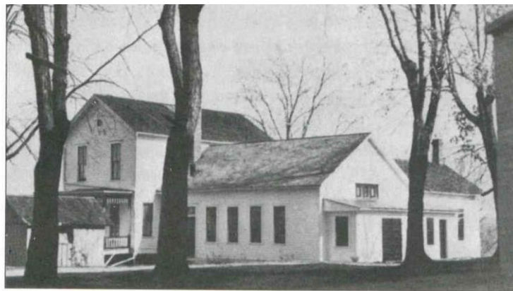
The third school building, erected in 1881, with the Sisters' House which was attached in 1882. The addition to the right of the school was built in 1908.
