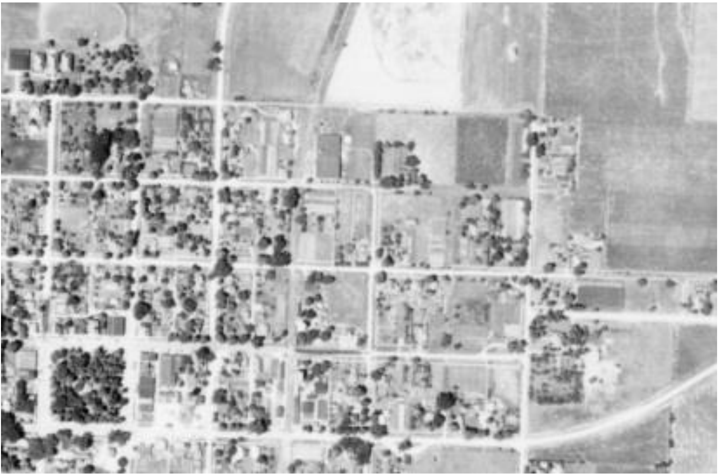
Northeast section – note that this picture was taken before the east side of the square burned in 1941
